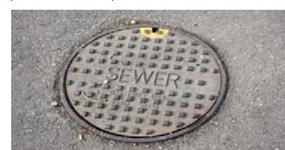
Repair ten leaking manholes on Messick Rd. Over the years wear and tear along with salt water from the tide coming over the road has caused some manholes on Messick Rd to be rusted. Resulting in the water tight seal to fail. This failure allows salt water and dirt to enter the sewer system. The DEQ consent order states that if we know of leaks we have to take action on repairing those leaks.
