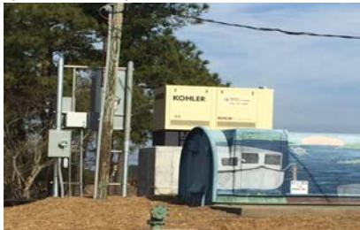
Installation of Back-up Emergency Diesel Generators at Pump Stations: Station #12 (Cedar Rd), #13 (Rens Rd), #5 (Wythe Creek), #16 (Dorothy Dr). These are listed in order of priority. Upon completion of this project, all sewer pump stations in the City will have generators. Upgrade of Back-up Emergency Diesel Generators at Pump Stations: Station #9 (Freeman Dr) and Station #14 (Roberts Landing). Due to age and wear, this equipment needs to be replaced.
