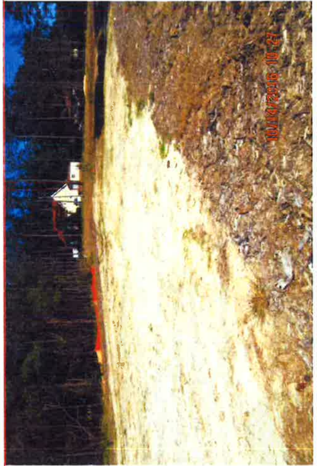
Drakes Landing - Before and After Photos - Below picture 10/14/16 - Above picture 10/28/16 - Site does not meet stabilization requirements in minimum standard 1 and minimum standard 3 of the Virginia Erosion and Sediment Control Handbook
