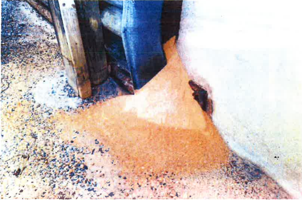
June-14-2017- Repair hole (outside) N corner of sand pile (covered).
