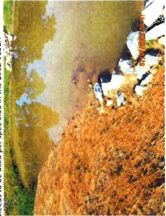
Top Right: Dirt bag for dewatering during pipe installation – Looks Great
