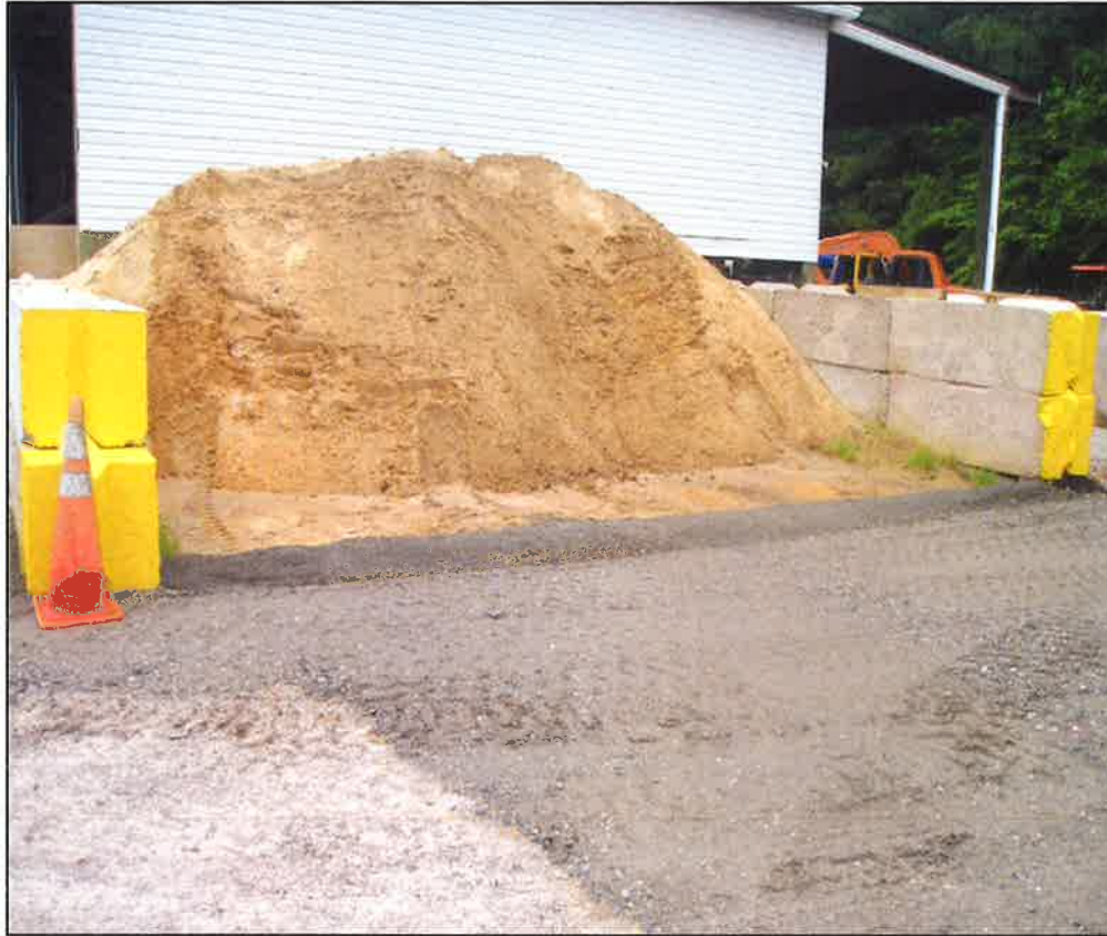
Figure 8. Premanufactured Block Containment
