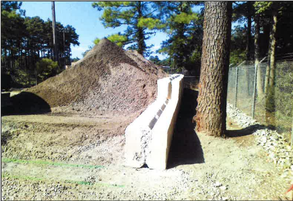
Figure 9. Rock Check Dam Against Perimeter Fence
