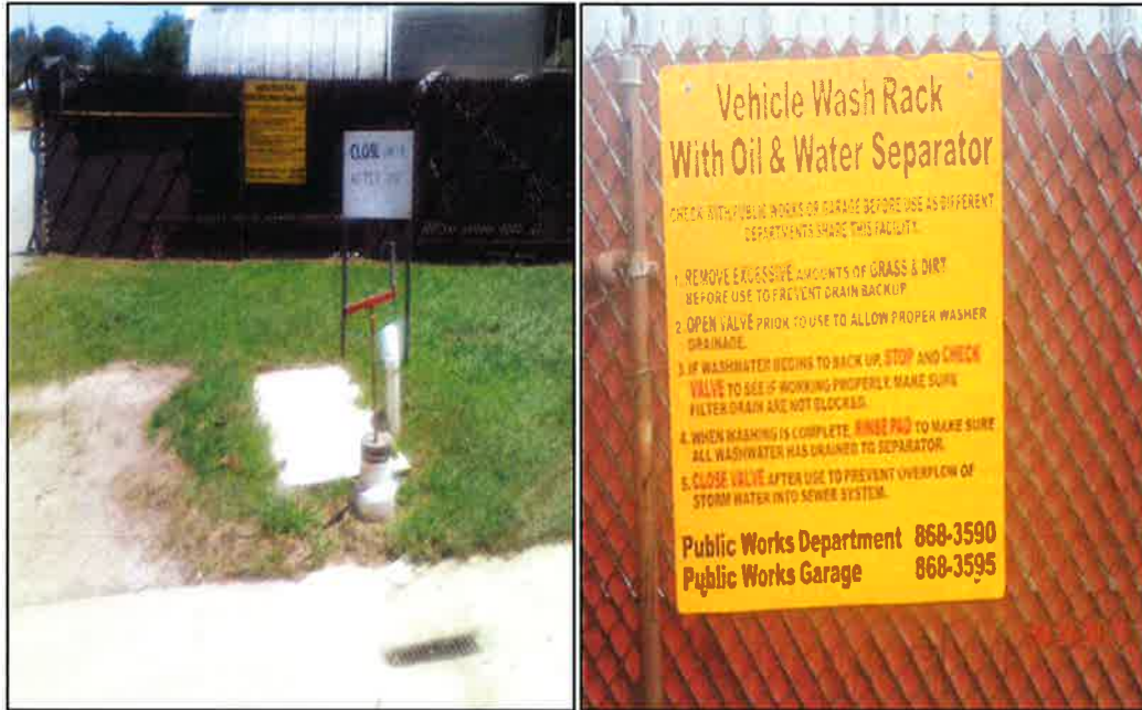
Figure 10. Wash Rack and Oil/Water Separator Area
