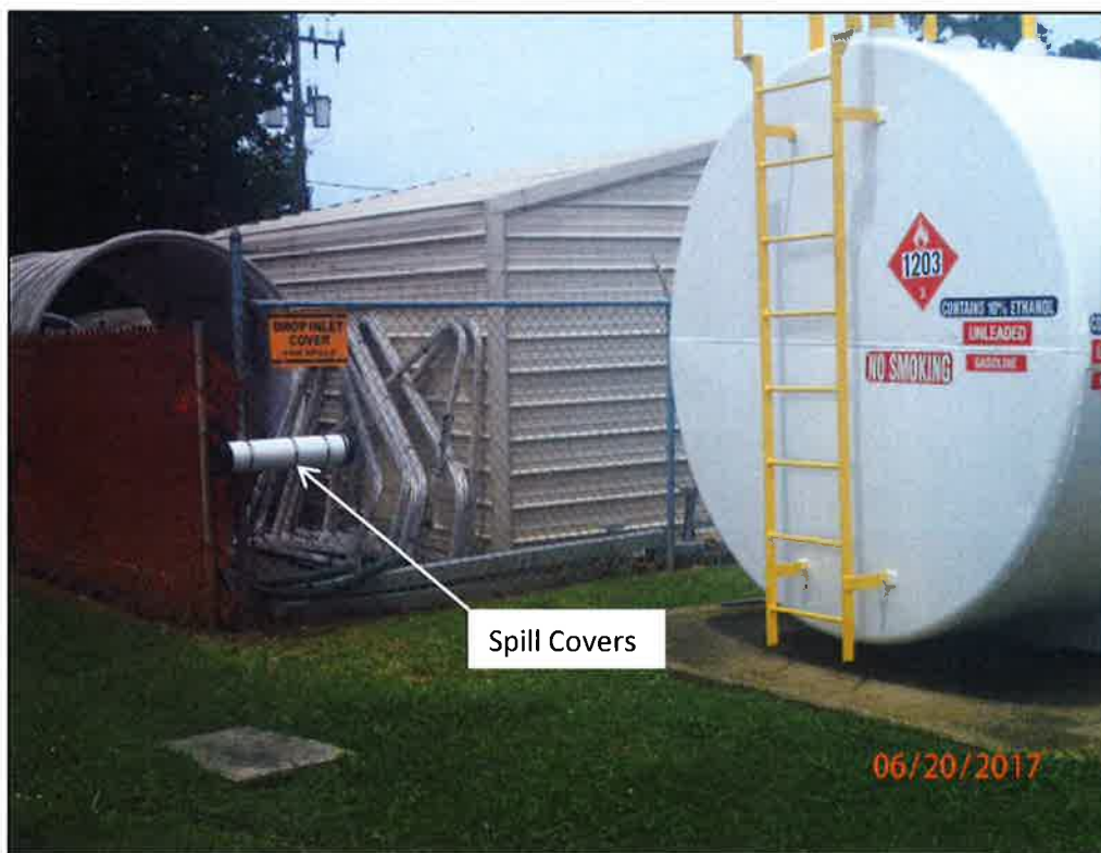
Figure 6. Drop Inlet Spill Covers
