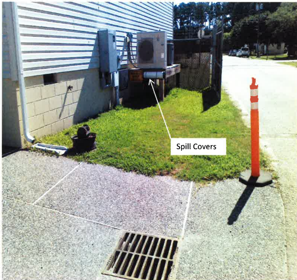
Figure 7. Drop Inlet Spill Covers
