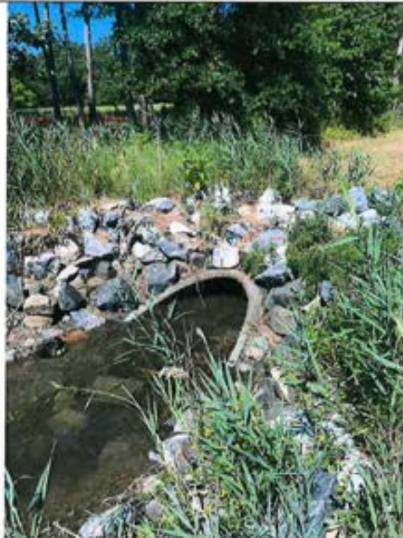
18. Outlet to Lyons Creek - Debris Present (Tidal)
