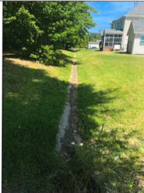
3. Temporary Berm and Temporary Low Flow Outlet Device
