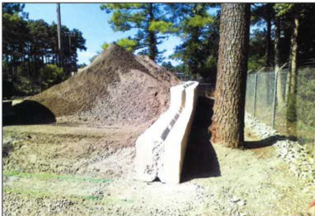
Figure 9. Rock Check Dam Against Perimeter Fence
