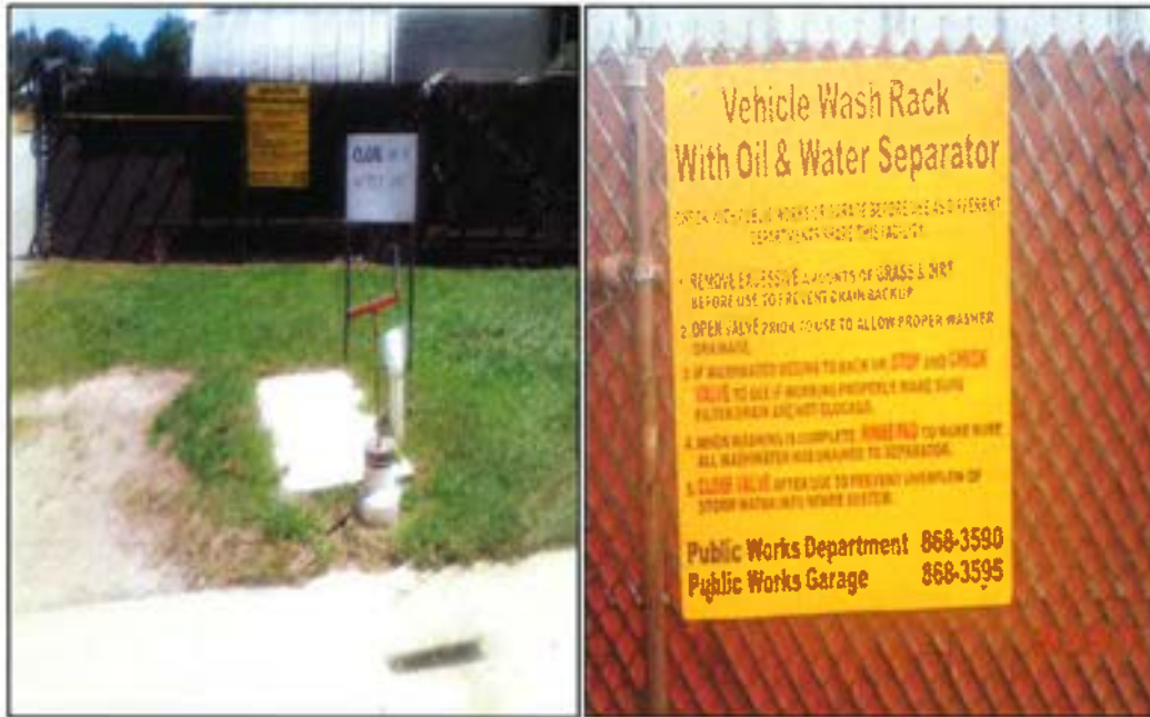
Figure 10. Wash Rack and Oil/Water Separator Area
