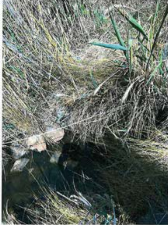
11. Inlet from Curb Gutters - Debris and Sediment Present
