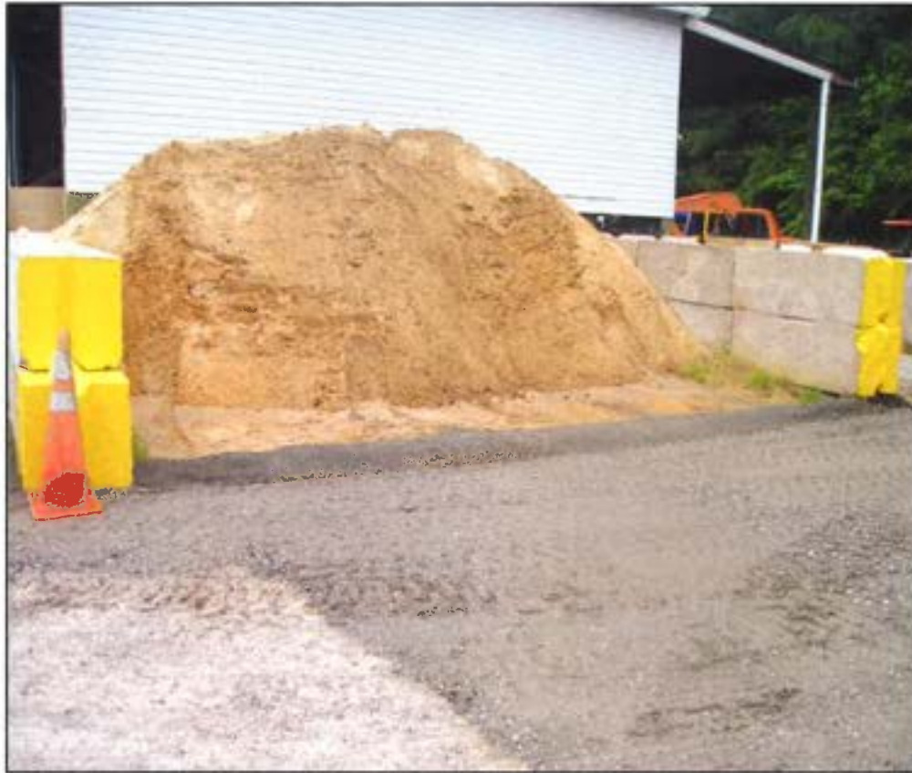
Figure 8. Premanufactured Block Containment
