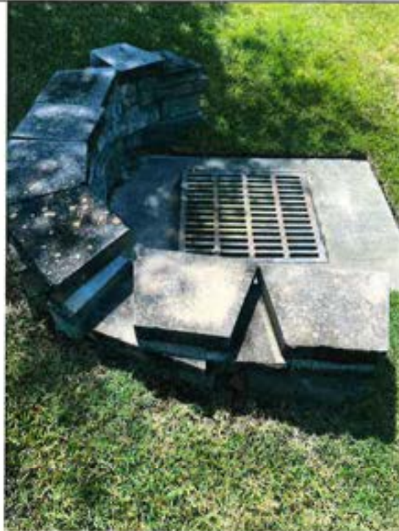
15. Temporary Low Flow Outlet Device
