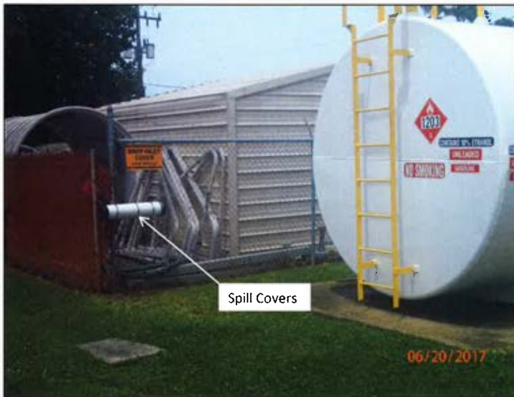
Figure 6. Drop Inlet Spill Covers
