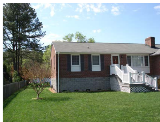
Elevated structure in flood-prone area of Poquoson. Photo courtesy of City of Poquoson.
